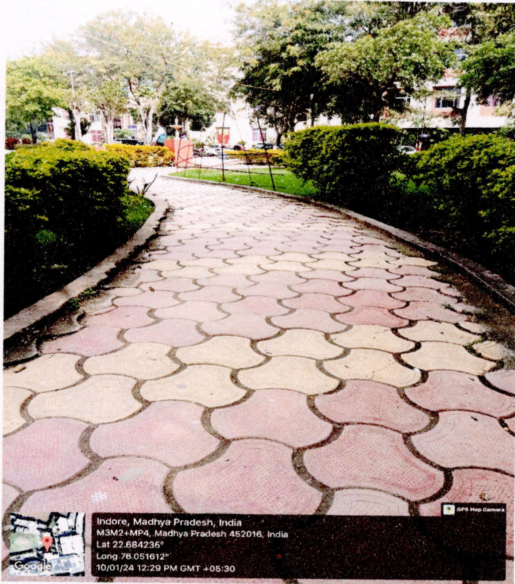
Photo: -Pedestrian Paved pathways
