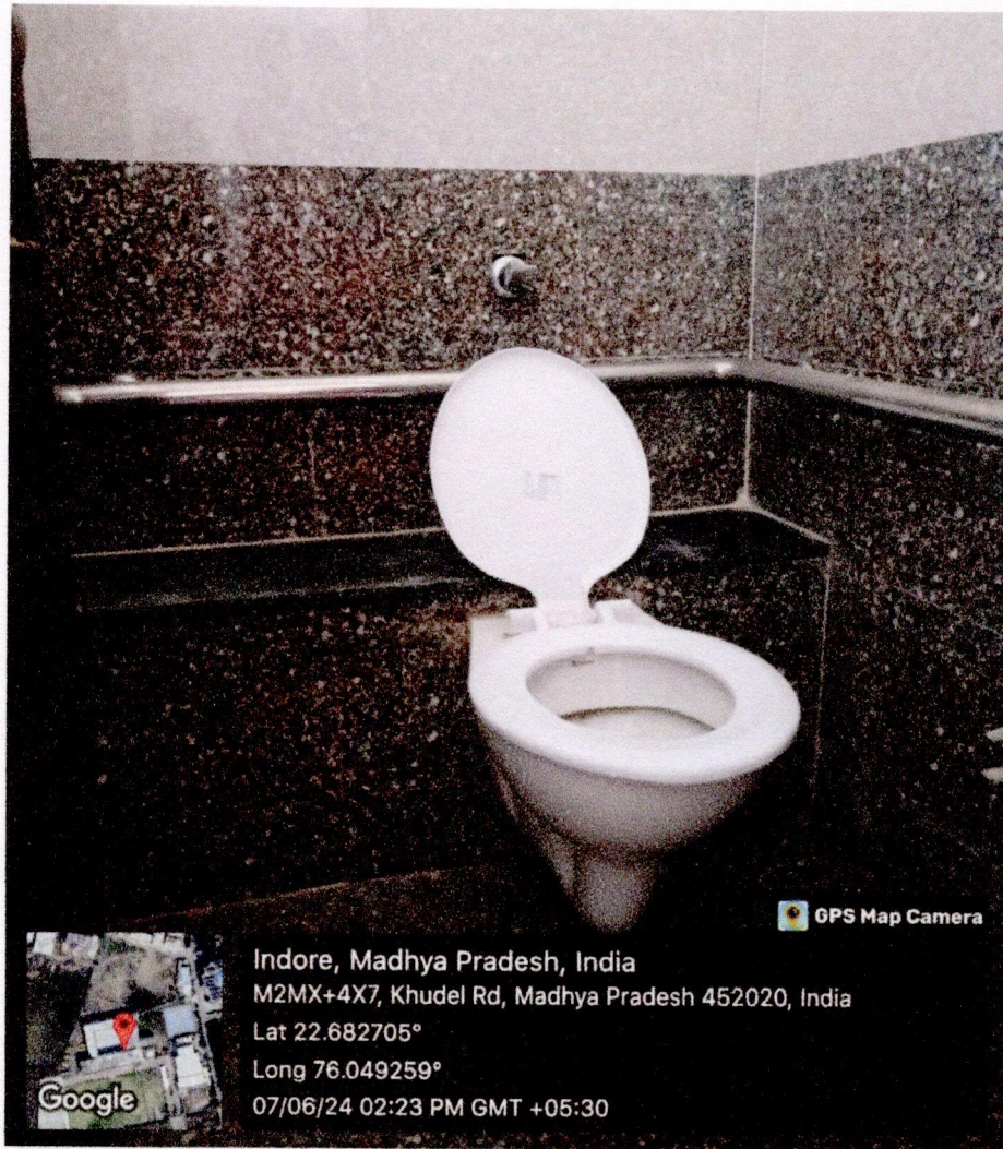
Photo:-Diyangjan friendly toilets with ramps & grab bar
